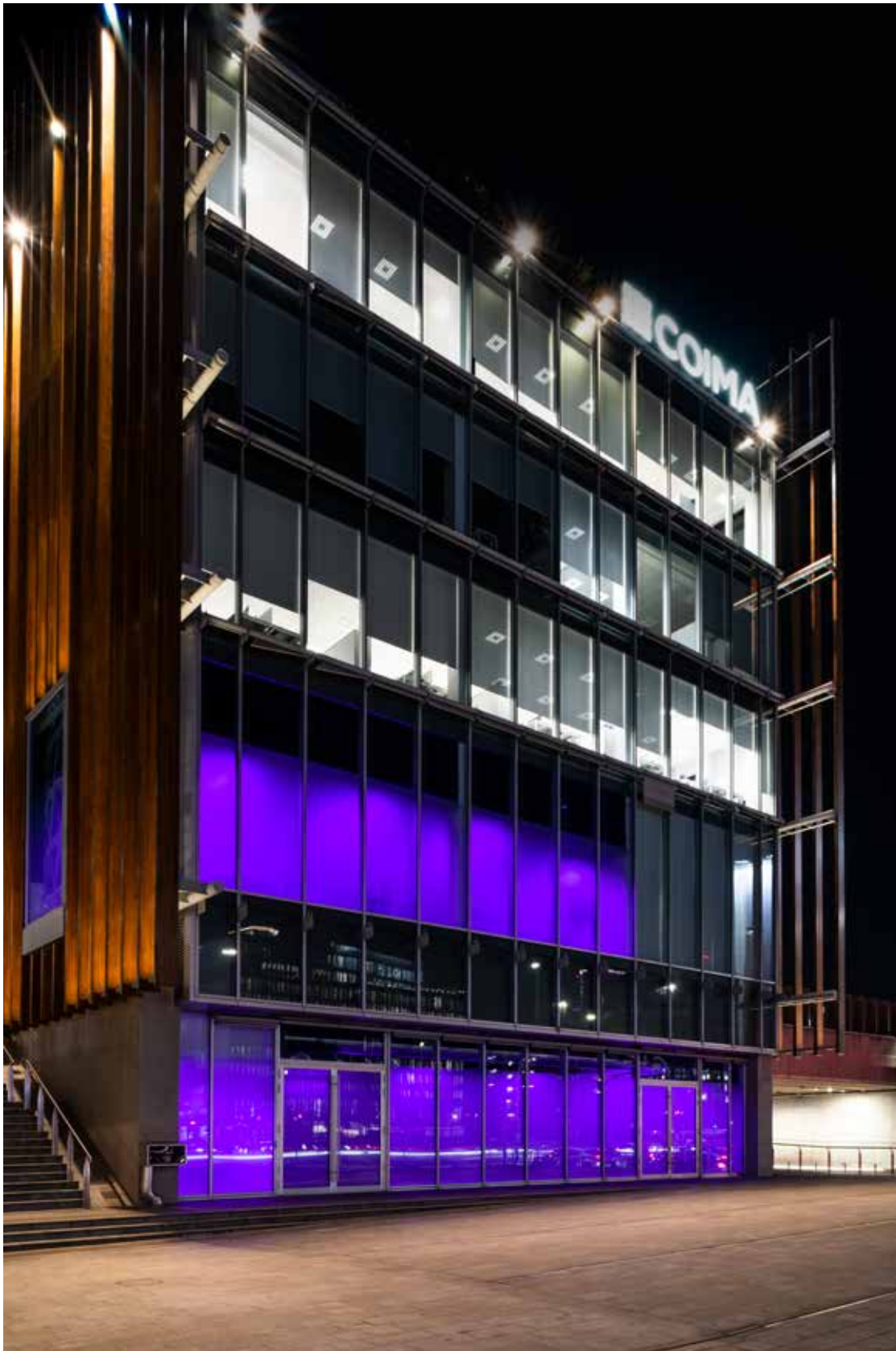
INTEGRALIS® installation HabiSmart by COIMA - Milan, Italy
